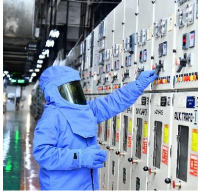
Using Arc Flash Suits to work on electrical panels
